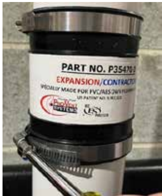
Tighten up the stainless steel bands 5
