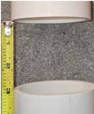
Leave a 2-3/4" gap between the pipes 1
