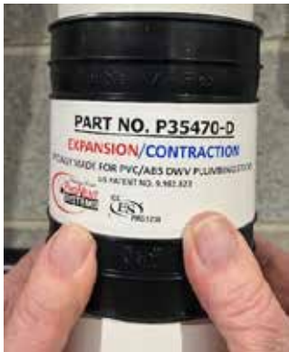
Roll back the two ends onto the pipes 4
