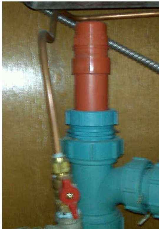
Mechanical Joint application
