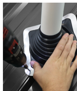
9. Secure flashing with screws
